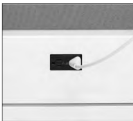
Duplex receptacles snap into raceway.
